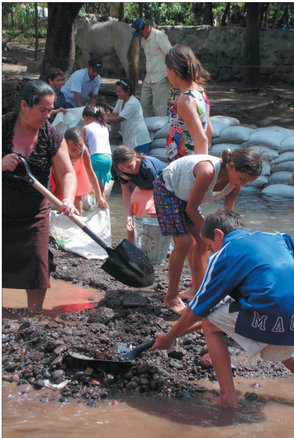
Flooding is a major problem for the people of El Molino Sur in Matagalpa, central Nicaragua. Here they are building up the local river bank, to protect their homes during the wet season.
