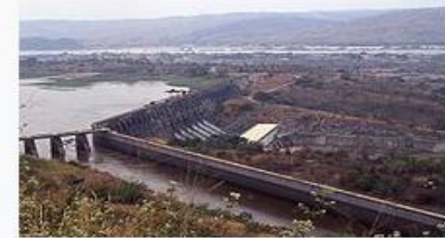
Inga I dam, with the feeding canal for Inga II in the foreground.
